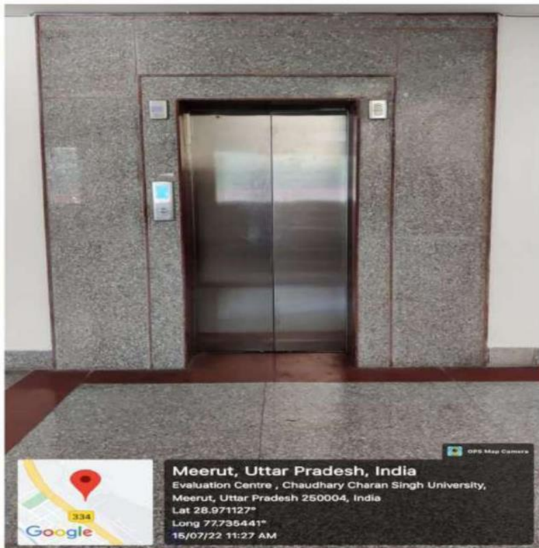
Lifts in Central Evaluation Building
